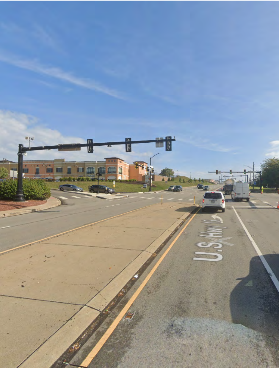
Some of State Route 19, image courtesy of Google Maps
